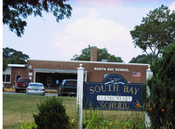
Figure 4 - South Bay Elementary School
